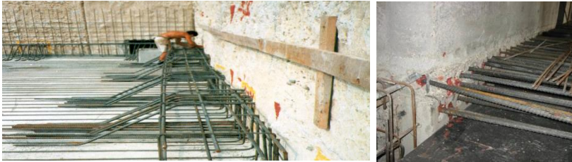
Connections of new slabs
