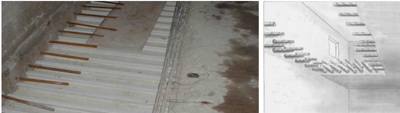
Close openings / slab enlargement
