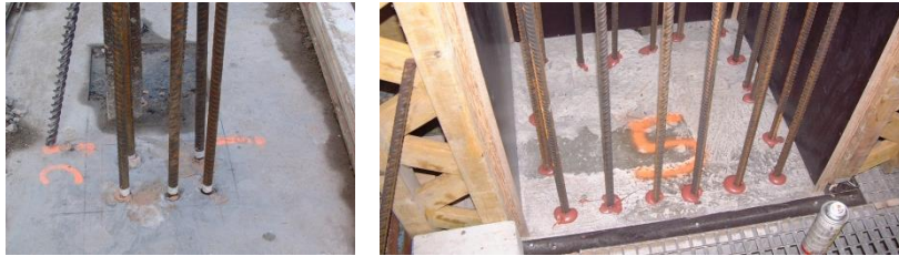
Connections of new columns
