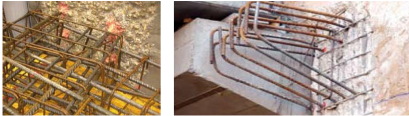
Connection of beams
