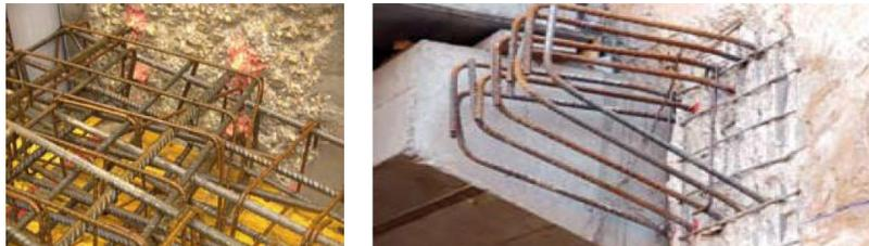
Additional / missing / misplaced rebars
